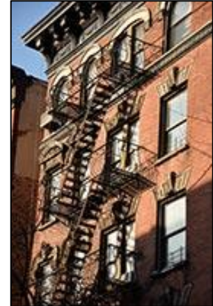
Source: Shutterstock This photo shows the upper three stories of a brick apartment building.
