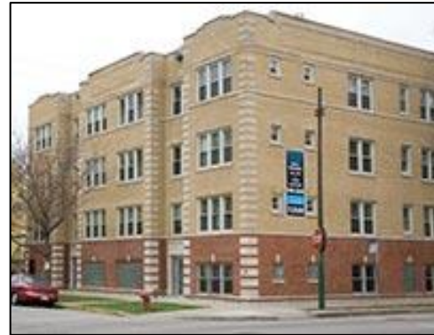
Source: Community Investment Corporation. This building is an example of a small multifamily property in Chicago. BMO Harris invests in buildings like this through the Community Investment Corporation loan pool.
