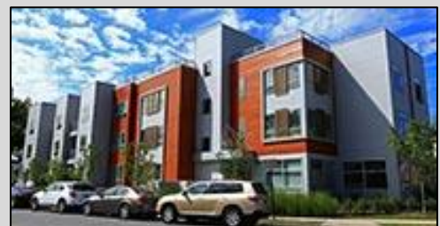
Source: Ronald L. Glassman for the Community Preservation Corporation. This 28-unit rental apartment building in Greenburgh, N.Y., received financing from the Community Preservation Corporation as well as private capital and public subsidies.
